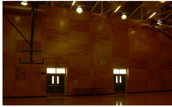
Gymnasium floor needs to be refinished.
