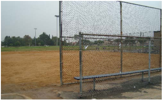
Softball infield and backstop are in poor condition.
