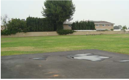
Minor ponding and flooding issues on campus.
